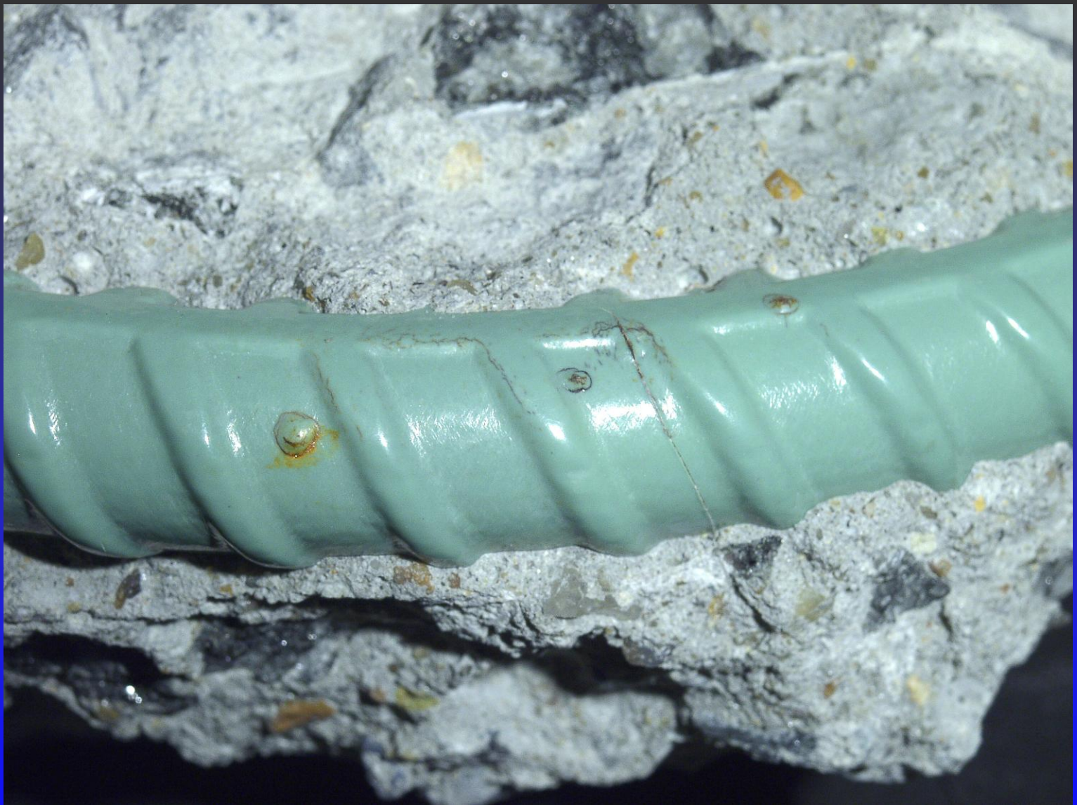
A Zn-Epoxy Coated Bar (1B) with a Cut Through Both Coatings. (Notice a corroded area under the coatings, at the top end of the cut.)
