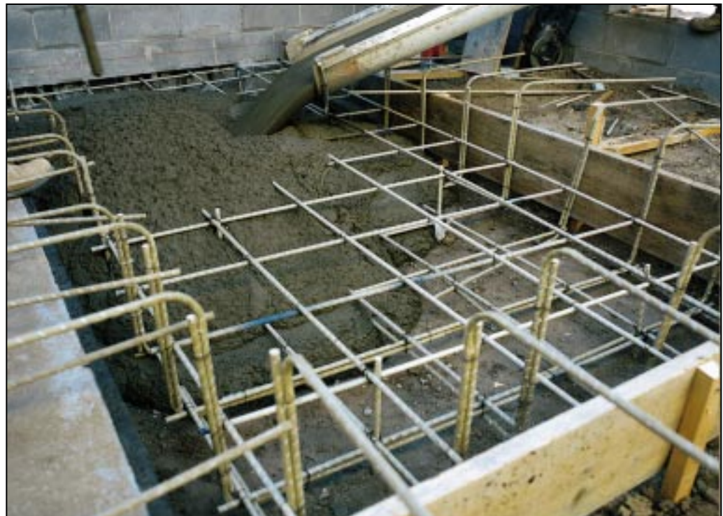
Glass-fiber-reinforced-polymer rebar can have twice the tensile strength of steel bars but are only one-fourth the weight. And because they contain no steel, GFRP bars won't corrode.
