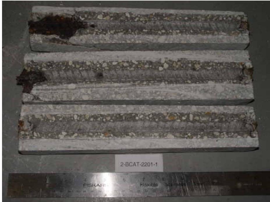
Figure 4.110. Photo. Trace of the upper rebars and corrosion products on specimen number 1-BCAT-2201-1.
