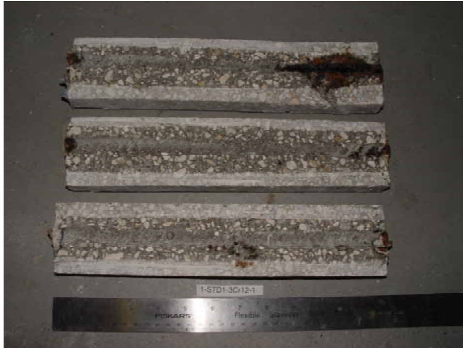
Figure 4.81. Photo. Trace of the upper rebars and corrosion products on specimen number 1-STD1-3Cr12-1.
