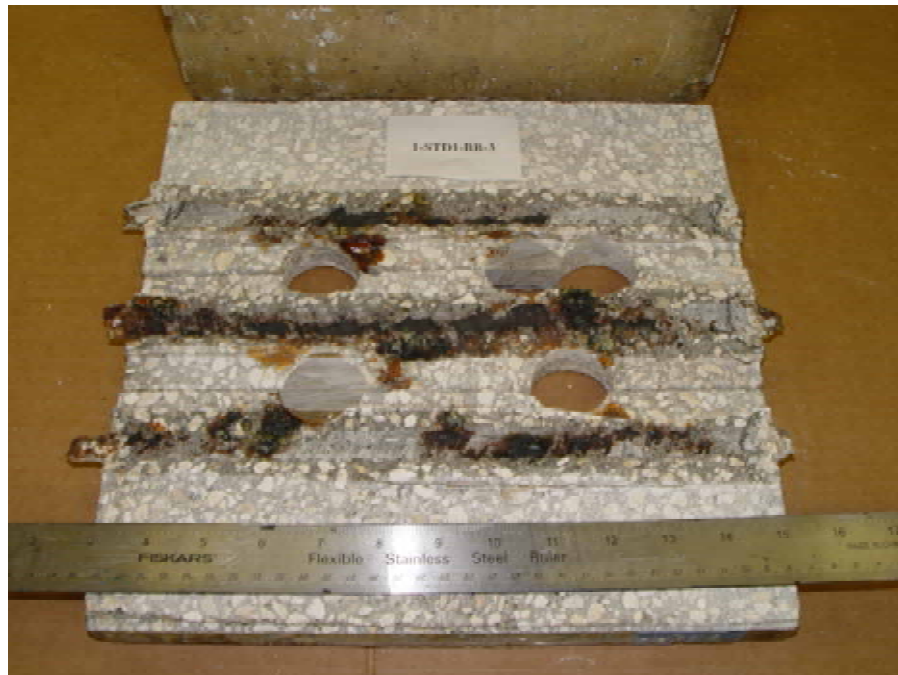
Figure 4.39. Photo. Trace of the upper rebars and heavy corrosion products on specimen number 1-STD1-BB-3.
