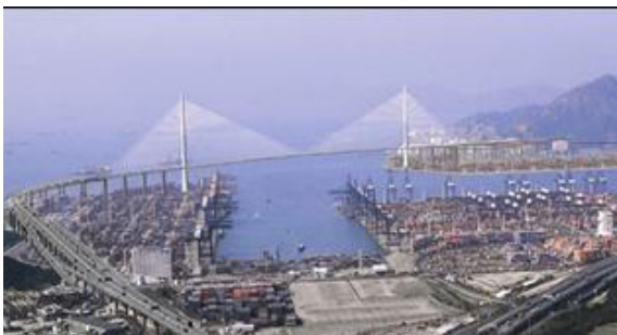
Figure 7-3: Stonecutters Bridge, Hong Kong. Pylons reinforced with SSR (1.4462) in the outer layer of the multi-layer of reinforcement
