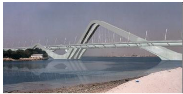
Figure 7-4: Sheik Zayed Bridge, Abu Dhabi. Lower part of supports are of reinforced concrete with SSR (1.4462) in the outer layer of reinforcement
