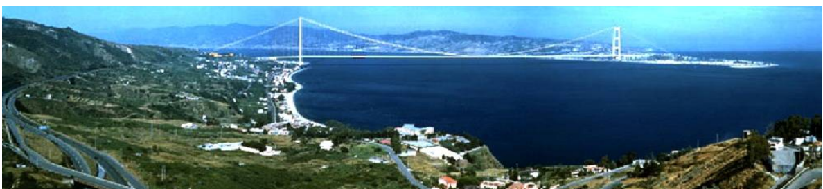
Figure 2-3: Messina Strait Bridge. Design service life is 300 years. Main span in steel is 3000 m. (Model Photo).
