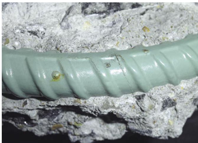
Fig. 15: The Zn/EC-1-1B bar recovered from a concrete block. Notice the four corrosion areas that ranged from 2 to 5 mm (0.08 to 0.20 in.) across and at 0 to 22 mm (0 to 0.9 in.) from the cut in the composite coating system
